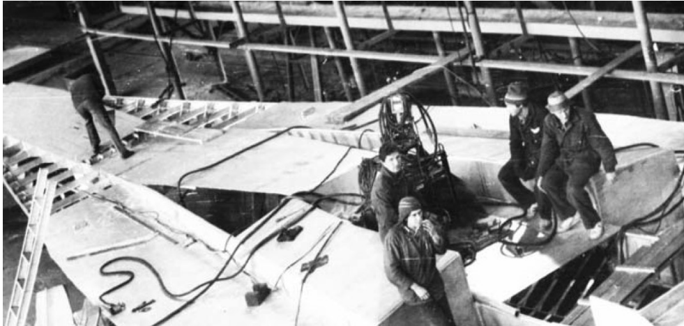
Alexei is inspecting something on the deck. On the floor lies the next deck panel ready for fitting. On the forward bulkhead you can see the triangular chainplate welded into the bulkhead. FAZ-05-080
