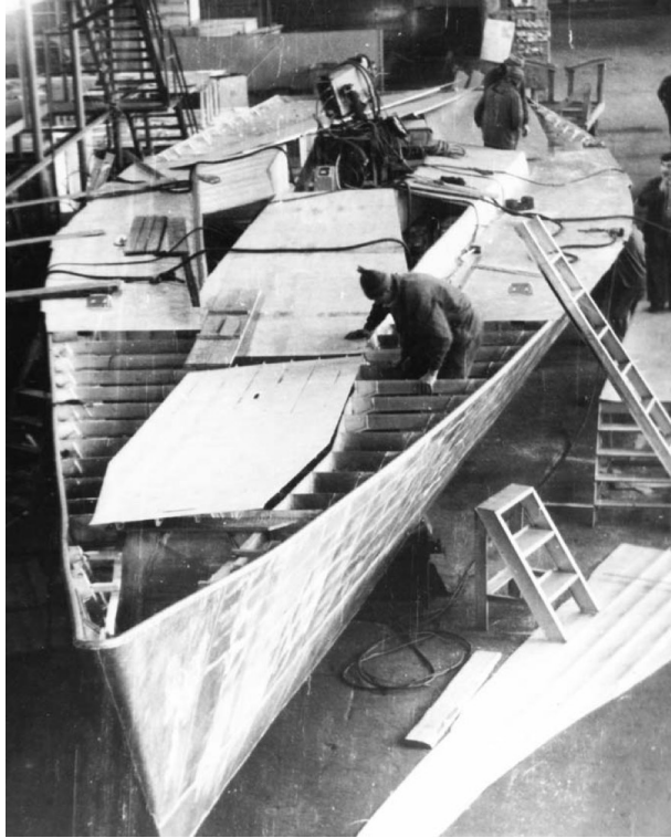
We are laying the deck panels. On the port side you can see the slots in the beams for the stiffeners. But those slots were never needed.
