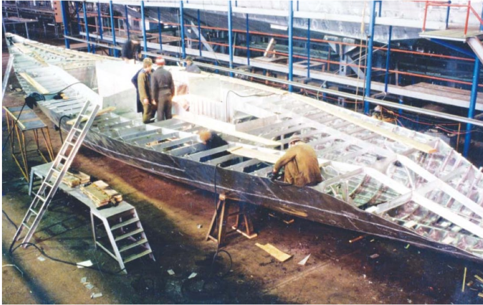
Planks are lying on the beams. We walked on them while there was no deck.
