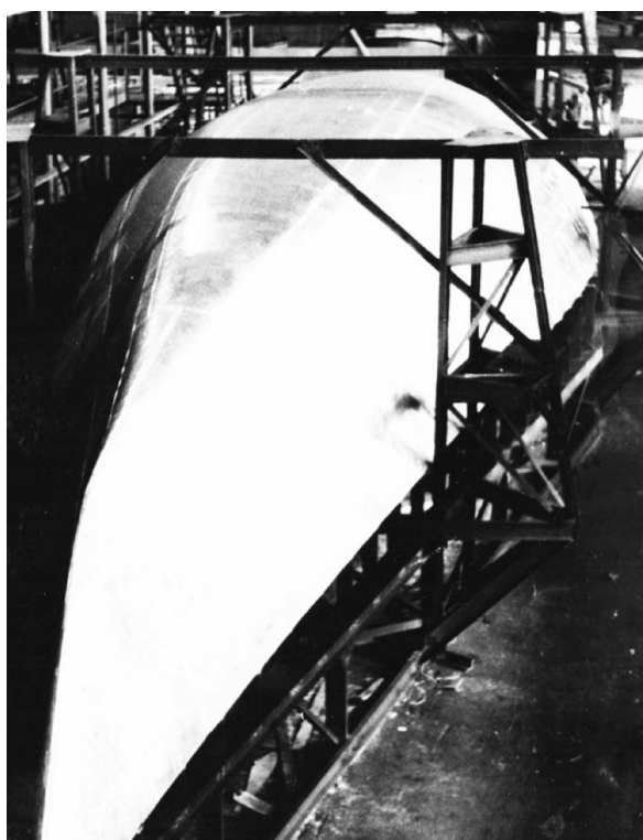
This is how the hull looked with the plating laid. It was hard even to fit the whole of it into the frame. The round black patch on the hull – nothing other than a mat to sit on. Sitting straight on the aluminium was cold.
