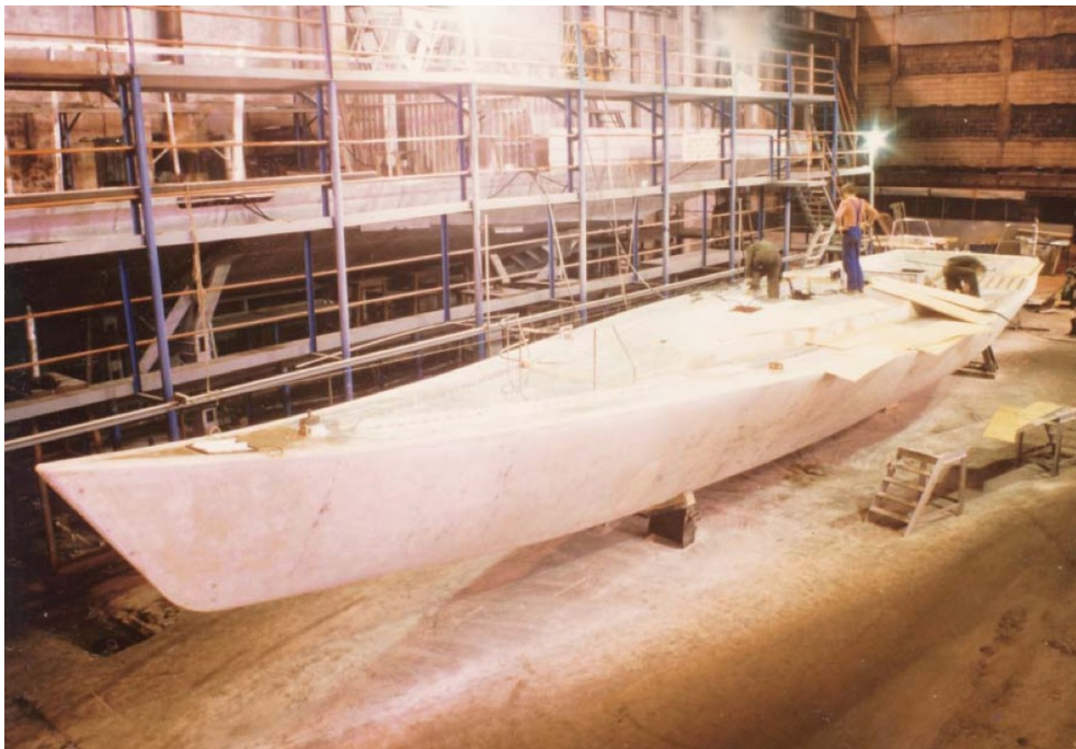
The hull is broadly finished. Getting it even to this state – took incredible effort from a lot of the lads. And all through not knowing modern methods in yacht building...
