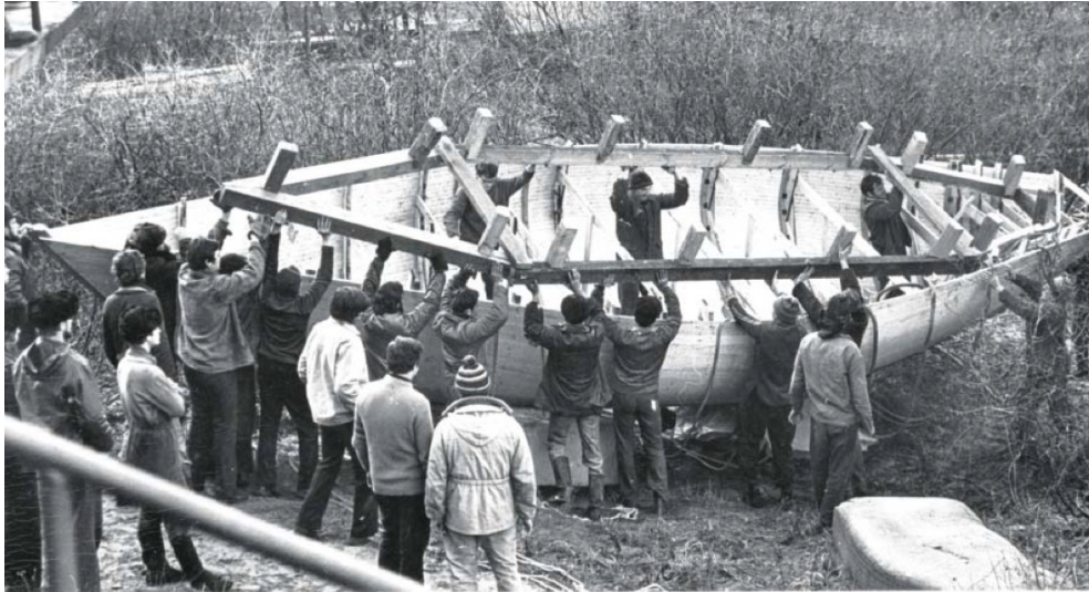
February 1979. Yura inside the boat. The main frames are already standing on the moulds and waiting for spring so they can be glued up.
