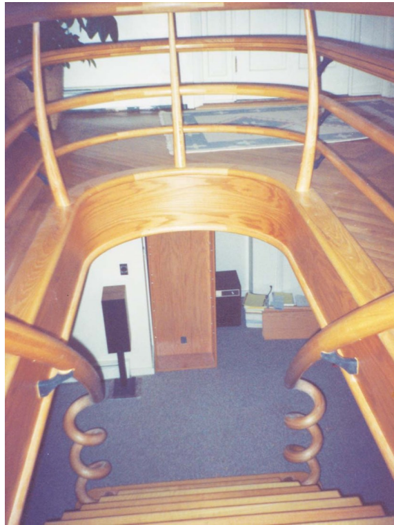
The top handrail – 76 mm in diameter. The handrail is continuous – it starts at the ground floor, rises to the first and comes back again to the ground floor. Material of the whole structure – oak.
